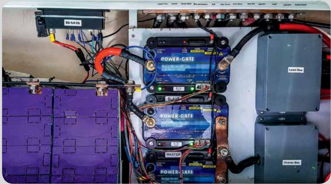
Lifepo4 batteries can give back about 80 percent of their rated amp-hours and not be seriously discharged. If you need 250ah of useable power, a 300ah Lifepo4 bank will be plenty.
